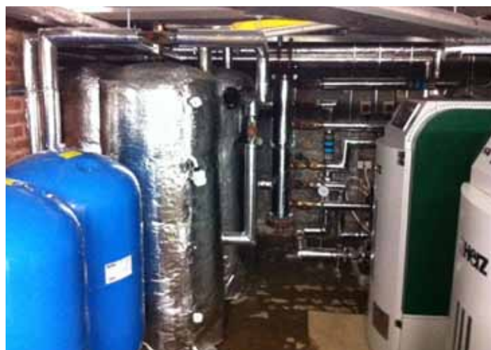
Figure 8: Biomass boiler installation
